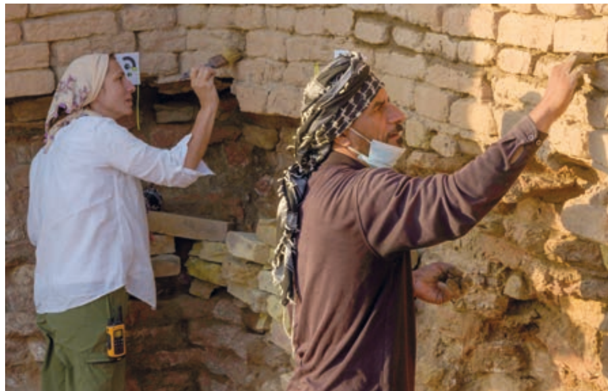
Conservation on the Sumerian bridge of Girsu.
